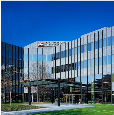
GENERALI Germany headquarter in Munich, Bavaria
